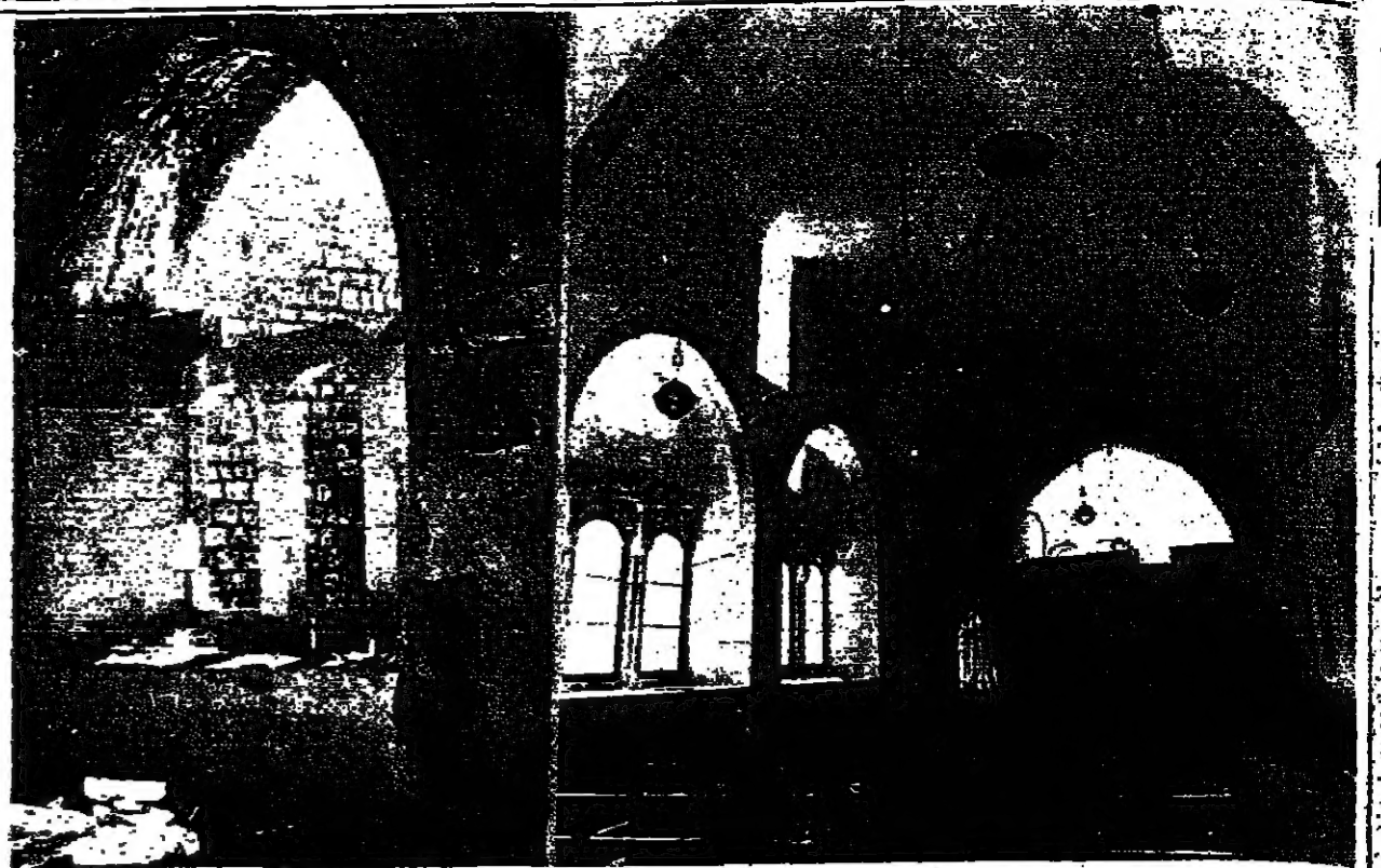
Four-hundred-year-old Yohanan Ben Zakhai Synagogue in Jewish Quarter of Old City is seen (right) as it appeared this week after restoration work that took four years. It is part of the Sephardi Synagogue complex which will be officially opened next month. Picture at left shows site in 1968, after four metres of rubble had been removed from synagogue interior.
